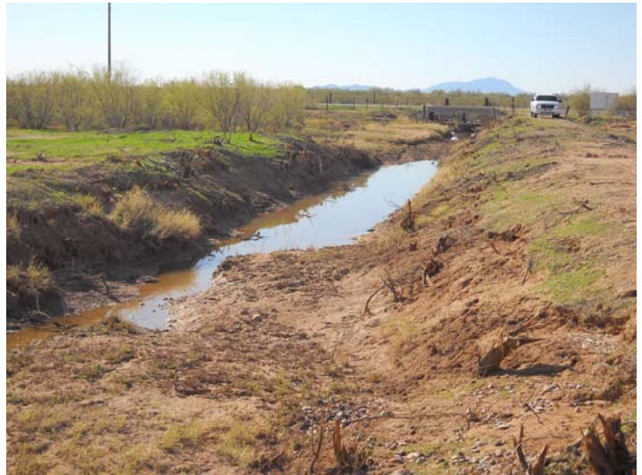
PHOTO NUMBER: 6 PHOTO DIRECTION: South DESCRIPTION: Outlet channel recently cleared of obstructive woody vegetation.
