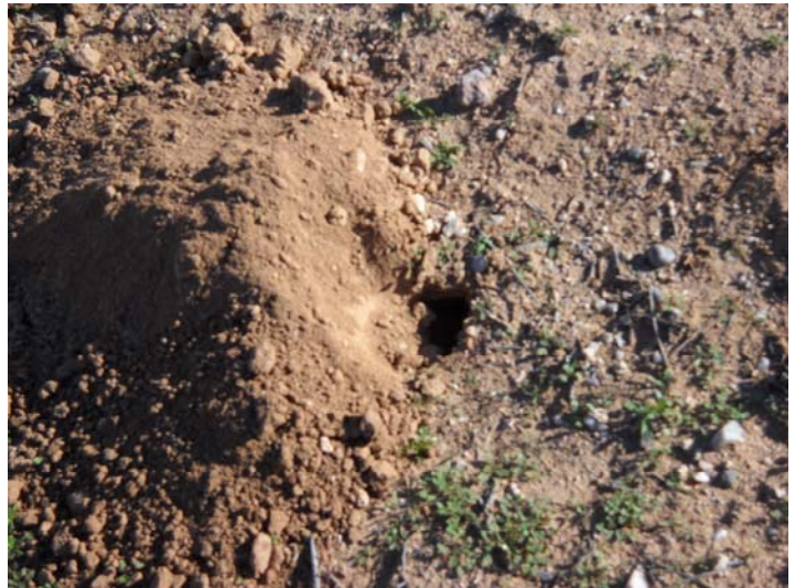
PHOTO NUMBER: 20 PHOTO DIRECTION: NA DESCRIPTION: Rodent burrow on upstream slope (typ.). Near inlet structure.
