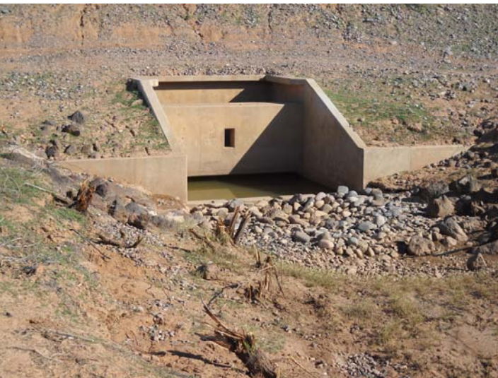
PHOTO NUMBER: 3 PHOTO DIRECTION: North DESCRIPTION: Outlet structure and baffle basin.
