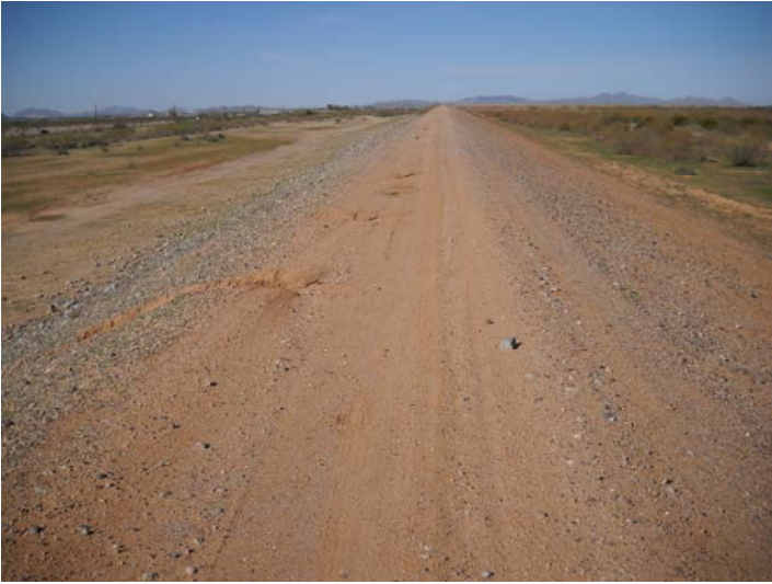
PHOTO NUMBER: 13 PHOTO DIRECTION: West DESCRIPTION: Crest of dam with sinkholes at cracks
