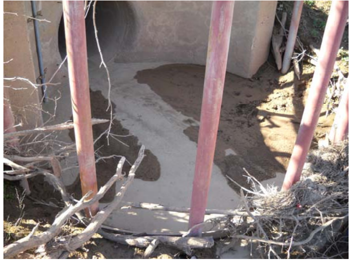
PHOTO NUMBER: 18 PHOTO DIRECTION: Southwest DESCRIPTION: Inlet structure and trashrack.
